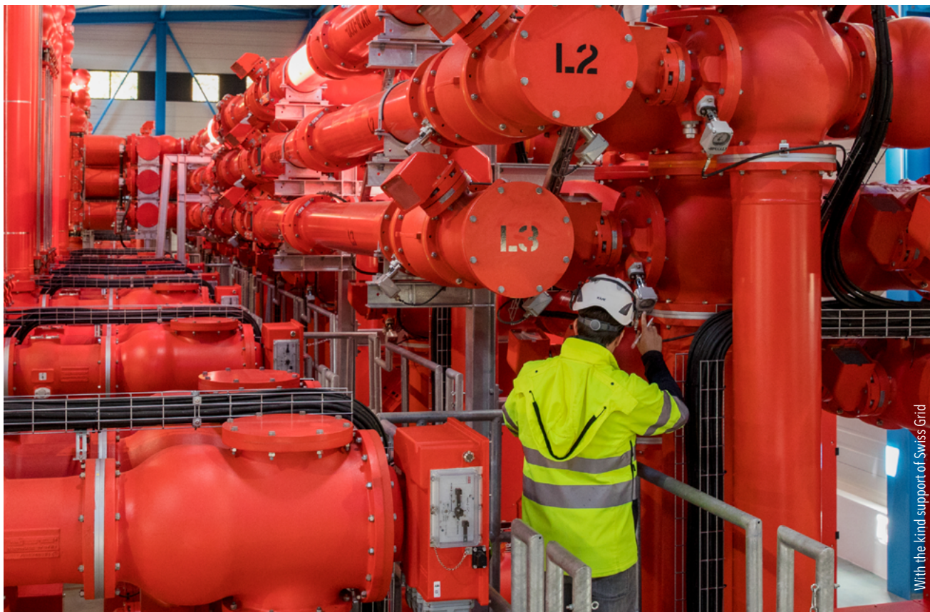
Compact, gas-insulated switchgear: Thanks to Trafag density monitors, the individual pressure chambers can be minimized.
